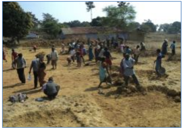
Implementation work under progress
