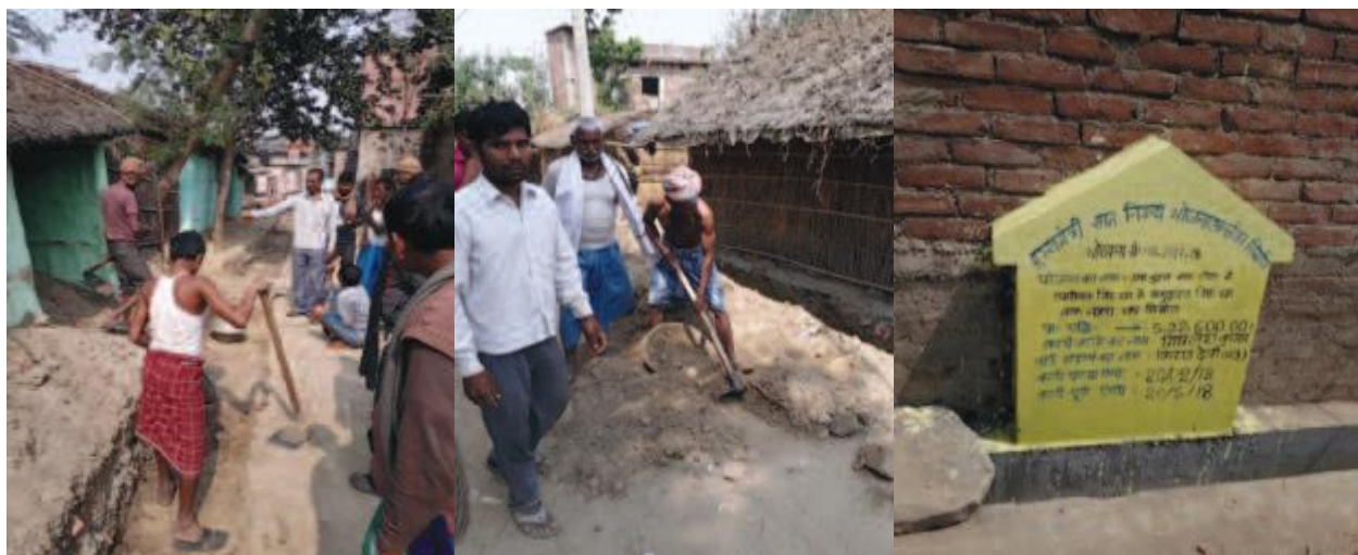
PCC ROAD AND DRAINAGE CONSTRUCTION UNDER SAATH NISCHAY YOJANA
