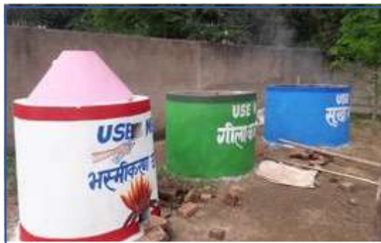
Incinerator, SWM unit and PWM unit in KGBP, Mahagama;
